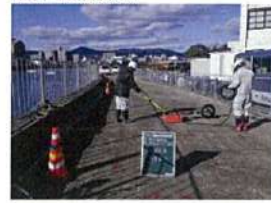
護岸空洞探査
